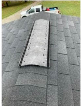
ridge vent installed over the porch attic space
